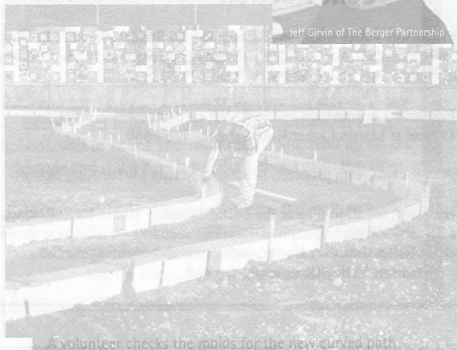
A volunteer checks the molds for the new curved path
