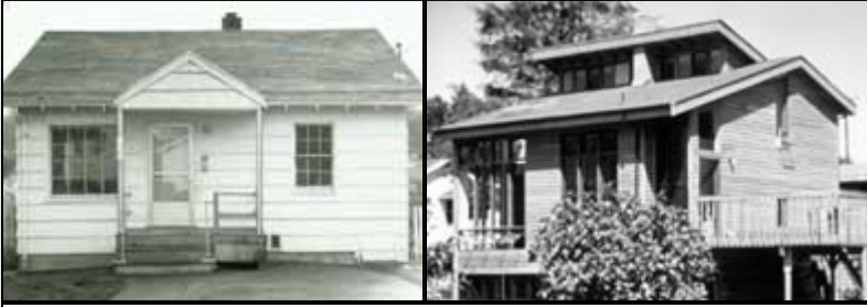
Before and After shots of "Solar I" built in 1980 in Madison Valley.
